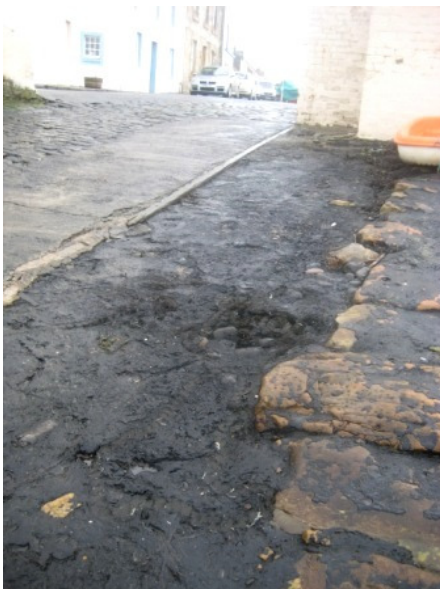
Heavy accumulation of tar on slipway associated with former boatbuilding.
