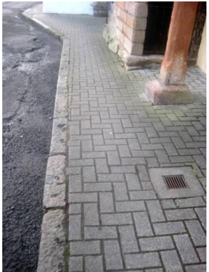
Modern concrete block pavements laid in a herringbone pattern.
