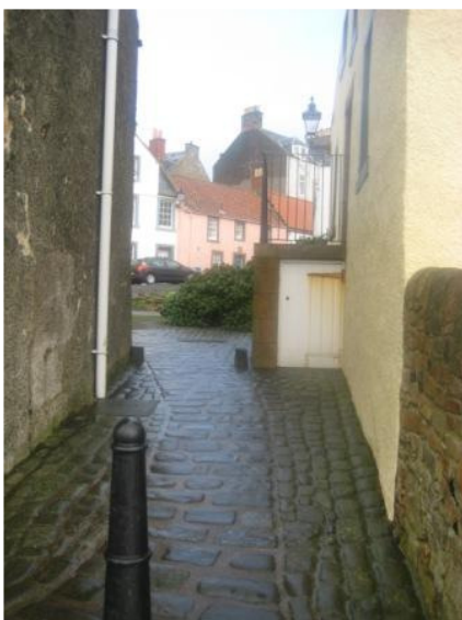
Re-laid sets and new bollard. Set in cement with much wider than traditional joints.
