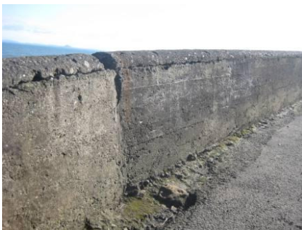
Shuttered concrete wave wall along West End.
