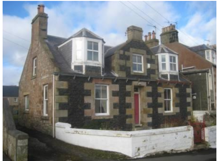
Unlisted 5 Braehead is a fine example of cherry corks whin rubble masonry skills.
