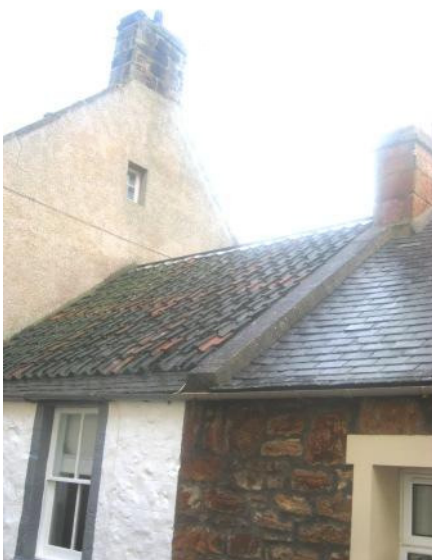
Typical mixture of traditional materials and finishes, adding diversity and interest. . Note unsympathetic PVC-u window to right-hand window and non-traditional brilliant white modern masonry paint left-hand cottage; and the rebuilt brick chimney head.
