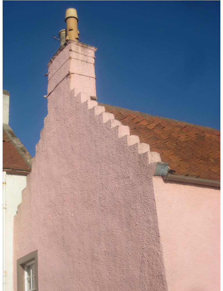
Pantiles, crow-stepped gable, skew-put and thackstone.
