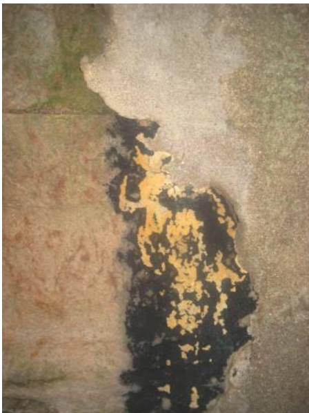
Seaward facing cottage wall with remnant of heavy uniform coating of black lime-wash with a white lime-wash later coating
