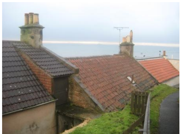
Modern concrete roof tiles far left roof.
