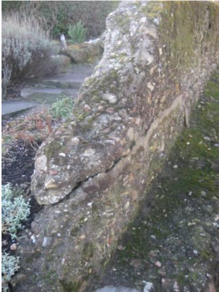
A damaged remnant of the wave wall to the west harbour pier of 1877 constructed using an early shuttered concrete technique
