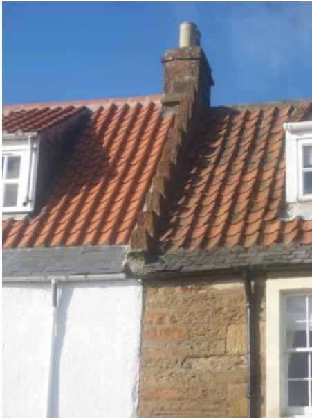
Contrasting old and new slate easing courses to pantile roofs.
