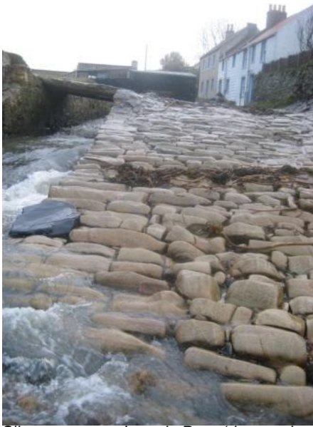
Slipway next to Inverie Burn (the nearby remains of what could be a former associated jetty or pier are revealed at low tide). The slipway is at risk of storm damage and loss. The mono-slab, Category B listed bridge in the background has recently been lifted and damaged by storm waves.
