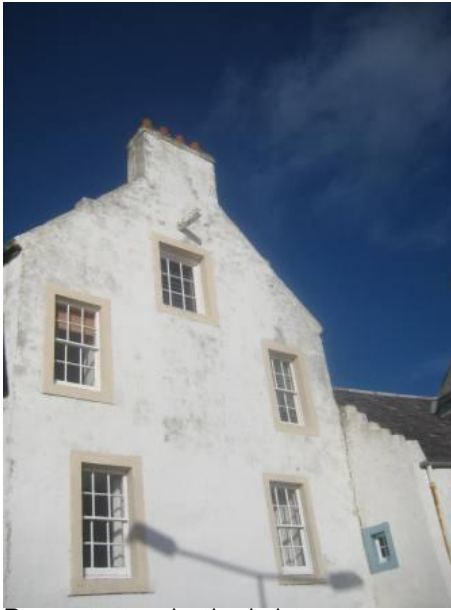
Rare extant projecting hoist gantry on the gable of 4 and 5 Mid Shore.
