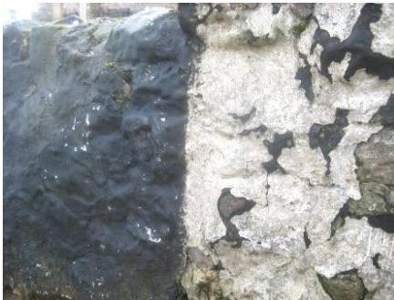
Rubble boundary wall painted in 'pitch' black and later over-coated with a lime-wash.
