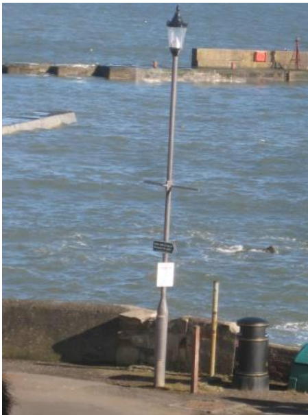
"Heritage range" lamp on a tall modern steel column and PVC-u waste bin.
