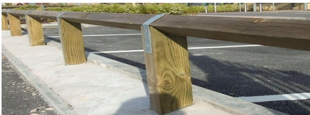
Picture1 – Typical shin rail with metal brace
