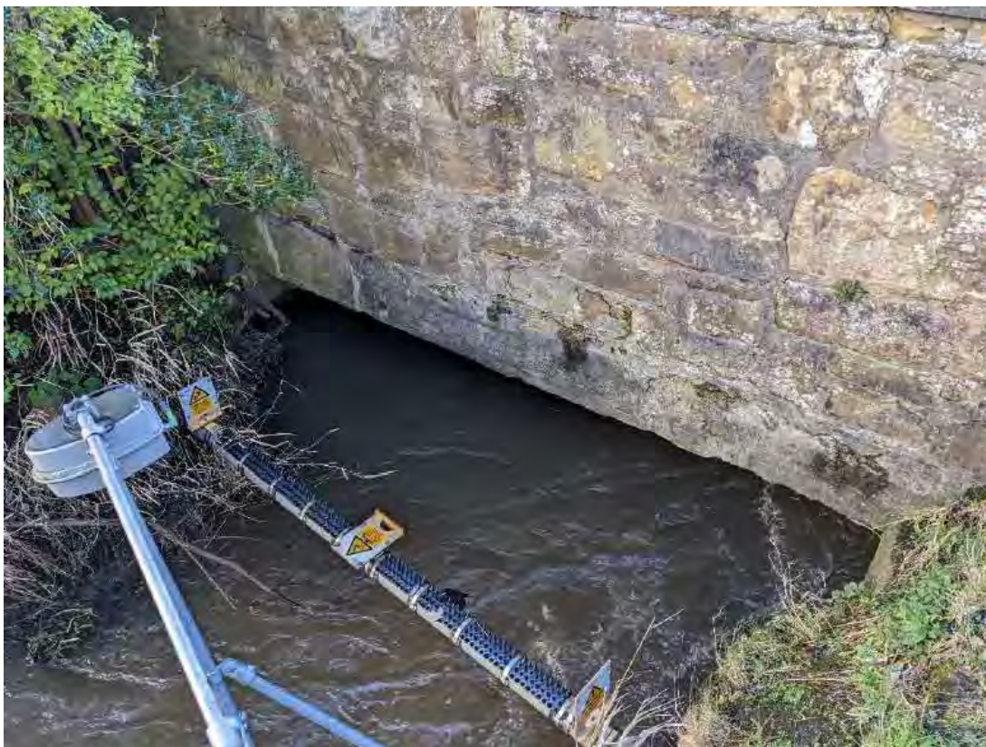
Figure 1 Upstream face of Cardenden Road Culvert
