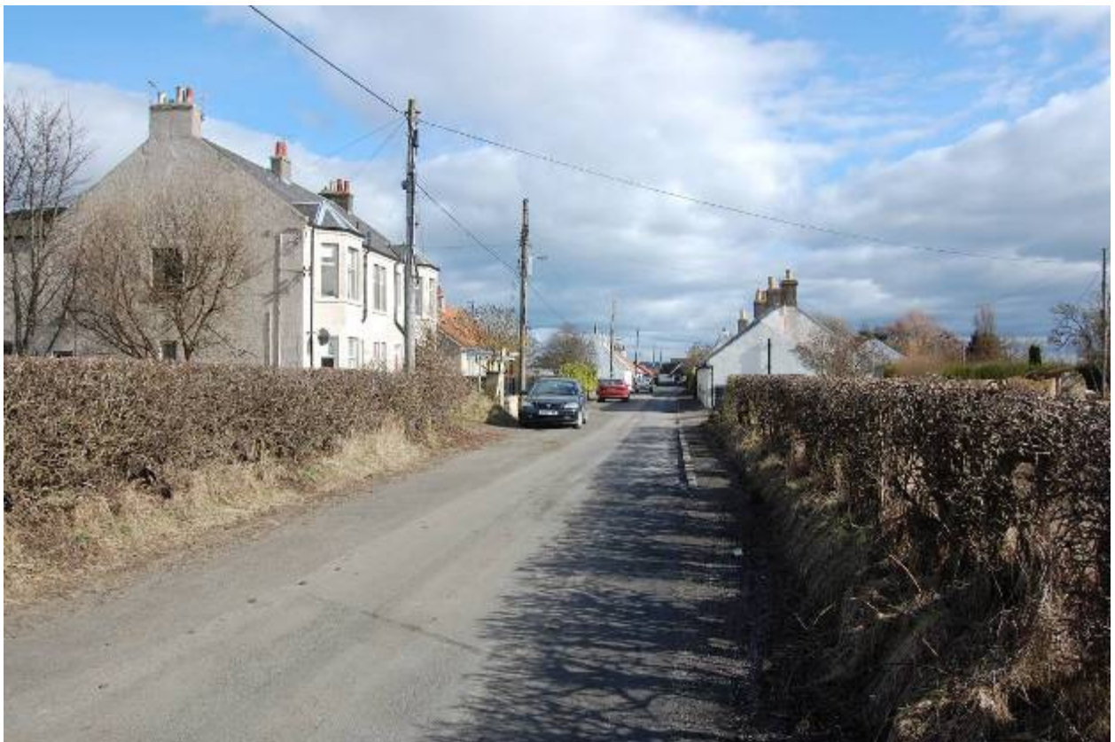
Contrast between building heights at the entrance to Pattiesmuir
