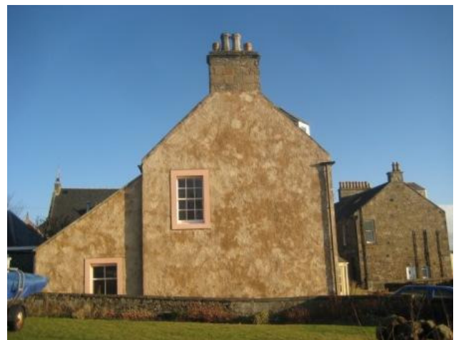
New traditional lime harl on 57 Main Street.
