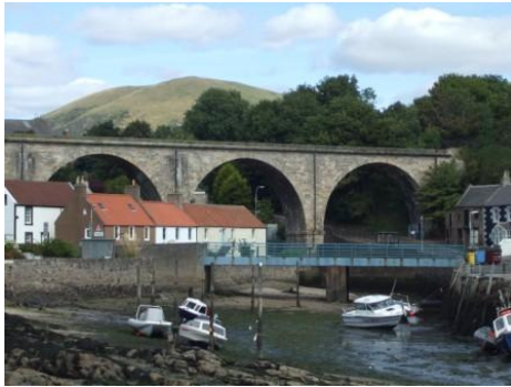
Old Railway Viaduct
