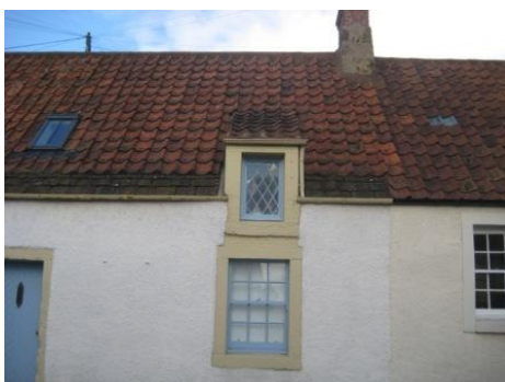
Pantile roof with slate easing course
