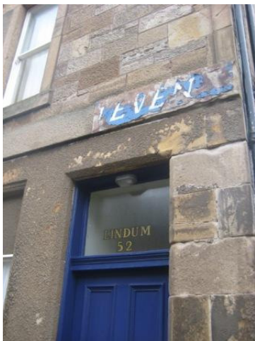
Cement slurry applied over ashlar at 52 Main Street
