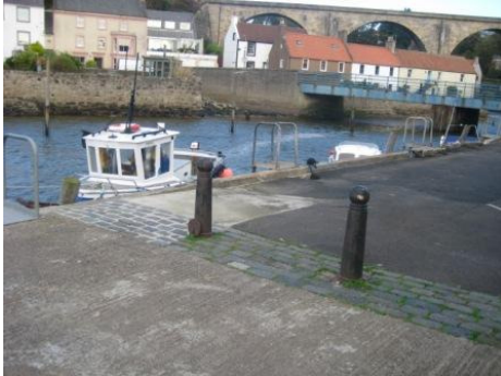
Modern bollards and surface treatments - harbour pier
