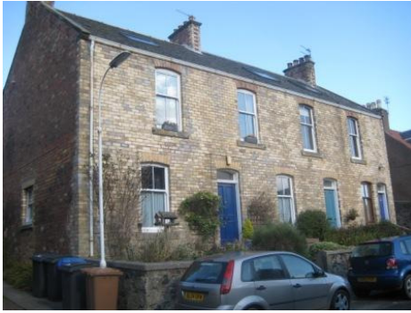
Brick masonry and Welsh slate roof
