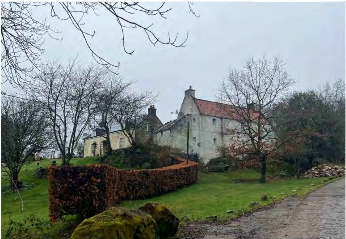
Figure 13 – Bath Castle with white masonry walls with stone walls and slate existing to Bath Farm Cottage
