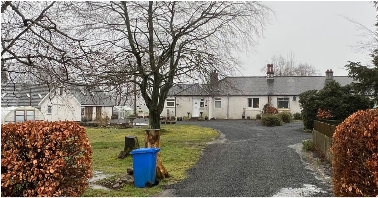
Figure 12 – White masonry walls and slate make up the materiality of Bogside Cottages. Further to this the semi-detached cottages have different coloured/ styled windows to one another.
