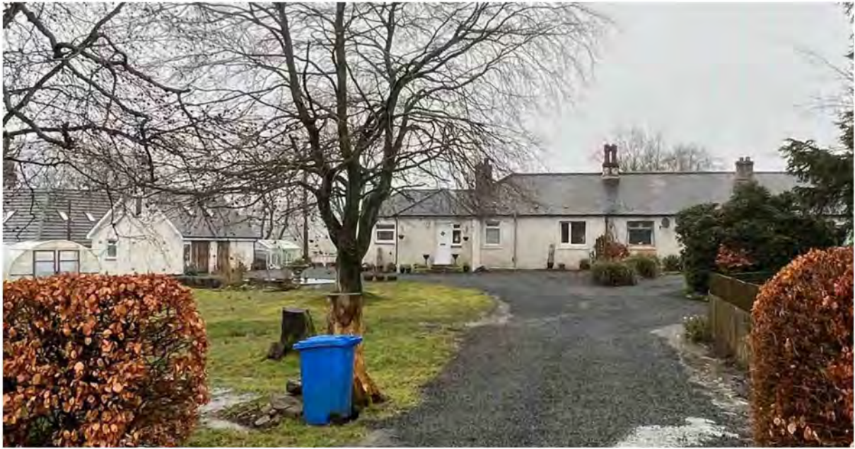
Figure 12 – White masonry walls and slate make up the materiality of Bogside Cottages. Further to this the semi-detached cottages have different coloured/ styled windows to one another.
