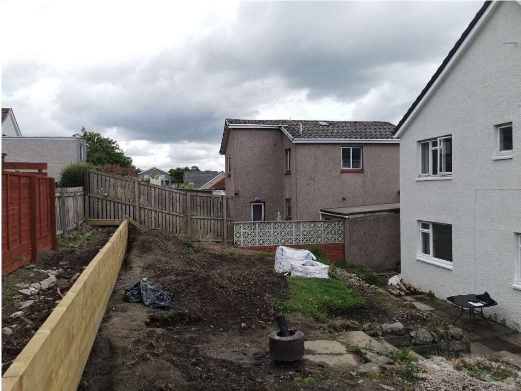
Site Photo - View to North-East
