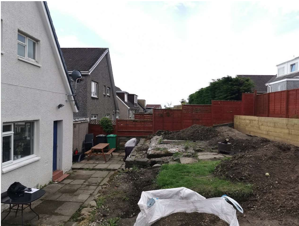
View to South-East
