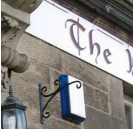
A sign screwed onto ashlar; the alarm box is insensitively placed on the front elevation – a side location would be better.
