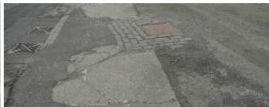
Well-detailed stone surround to inspection chamber set in various patches of asphalt
