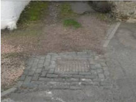
Church Lane/Church Place, showing a mixture of patch repairs in asphalt, pink gravel and natural stone paving
