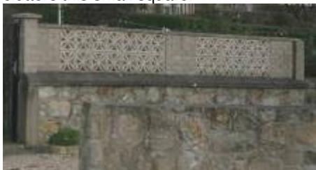
Concrete, off-the-shelf walling erected on top of a traditional rubble wall.
