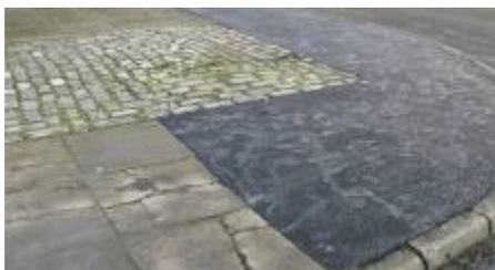
Recent asphalt near good quality stone setts and broken concrete paviors
