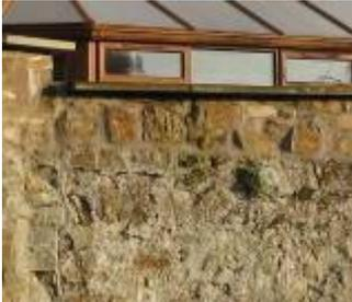
Concrete cope to rubble wall; cement pointing and unsympathetic repair
