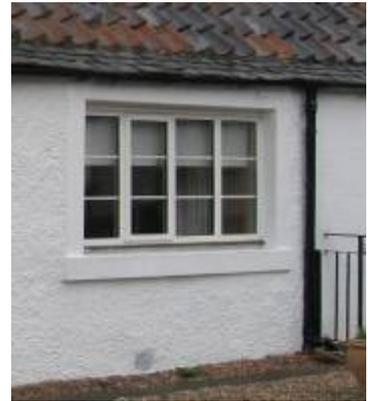
A range of inappropriate replacement windows, not matching original opening sizes, materials or design.
