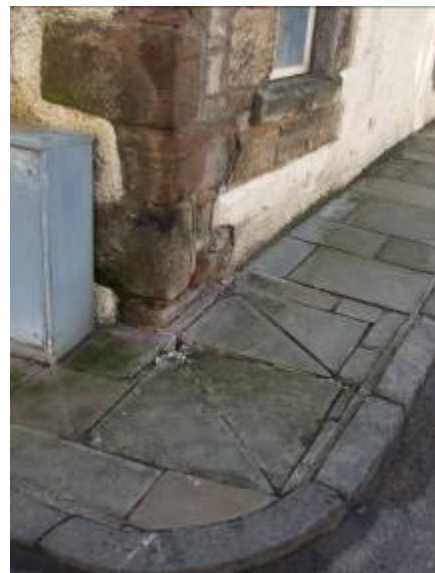
Yorkstone paving detail Main Street - 2009.
