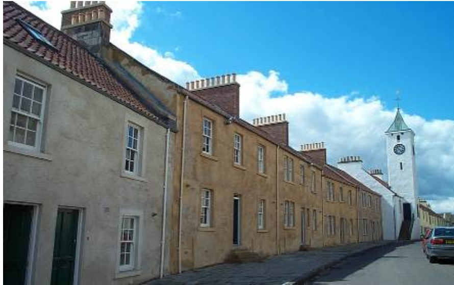
Front Elevation: South side of Main Street - 2001
