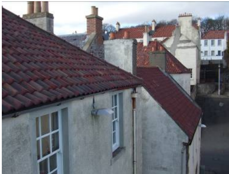
Roofing and Chimney Details, Burns Wynd – 2009
