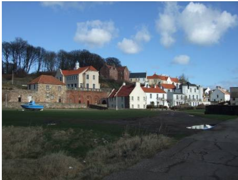
View of Coxstool and Belvedere Hotel across infilled inner dock - 2009.
