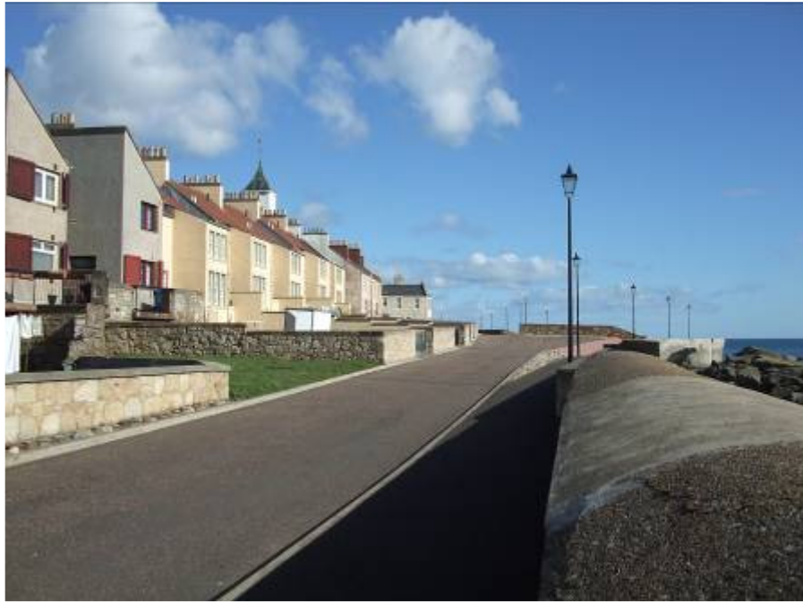
The Coastal Footpath and Coastal defence works looking east – 2009.
