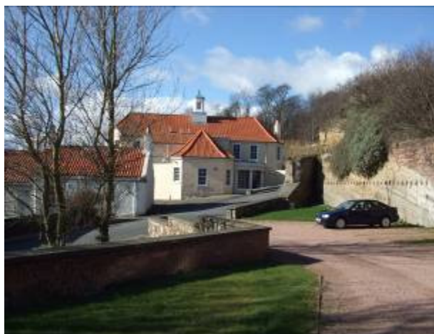
Windows boarded over on the Belvedere Hotel - 2009
