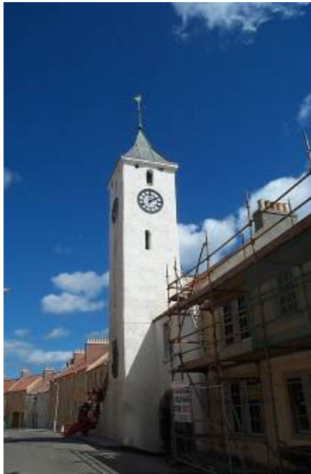
The Tolbooth and the flanking terraced houses during renovation in 2002-3.
