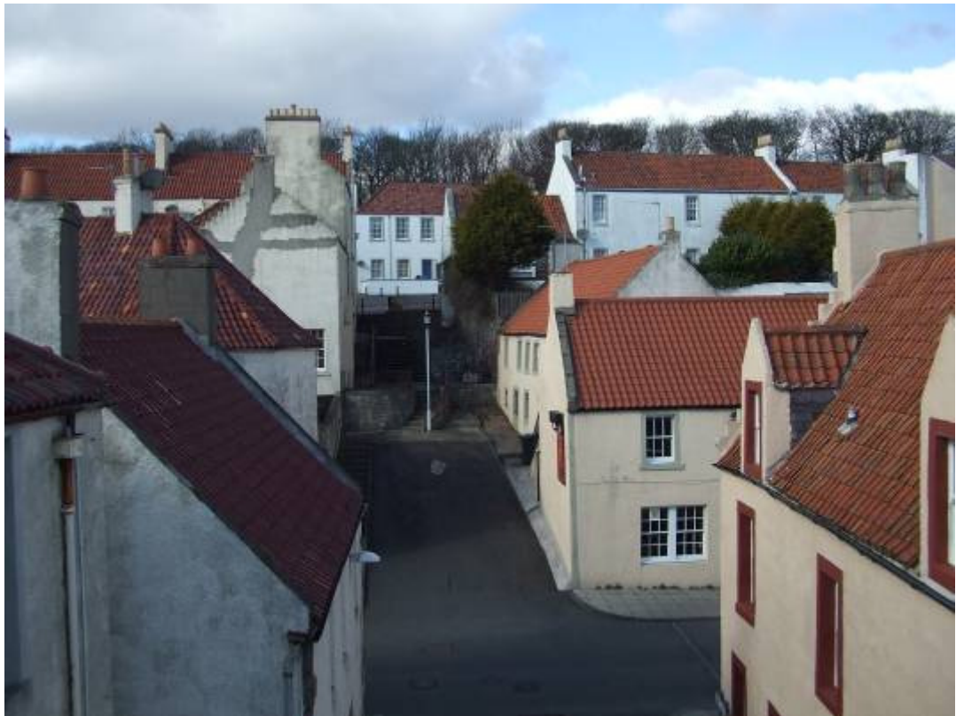
Rooftop view taken from the foot of Burns Wynd up towards The Cross - 2009.
