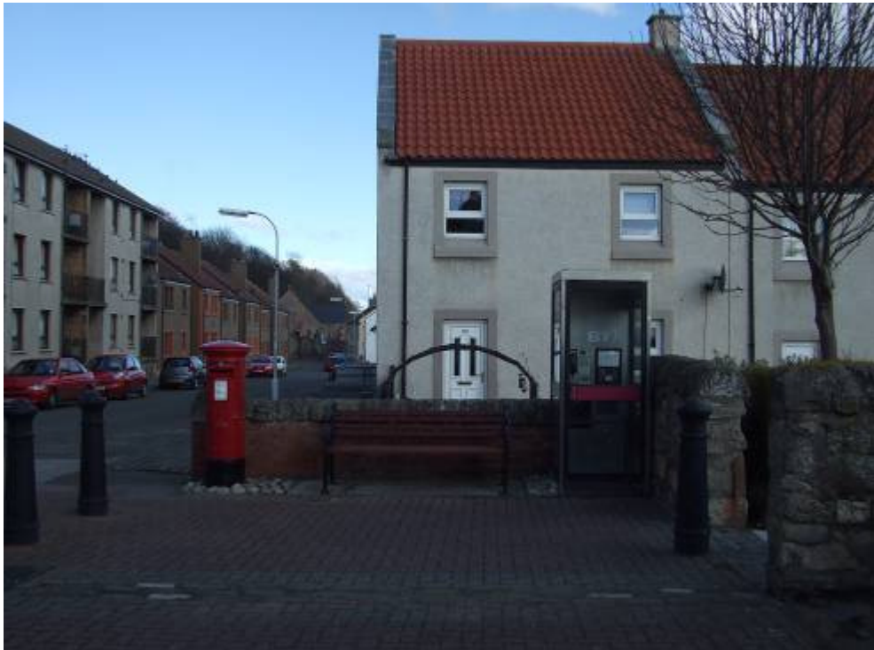
Poor quality public realm on Main Street. The 1980's phone kiosk, UPVc doors and windows and satellite dish erode the overall quality of the area.
