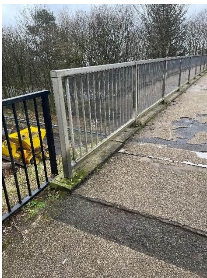
Footbridge crossing with Perspex panels
