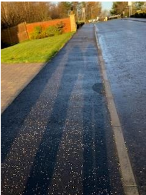
Lochtyview Way to roundabout
