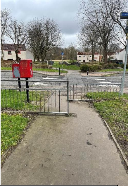
Crossing at Mar Drive
