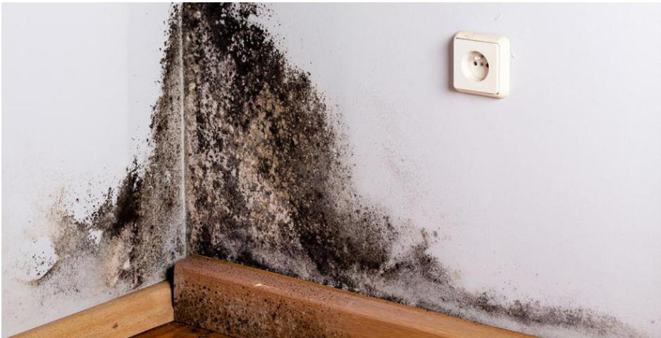
Penetrating damp is where water finds its way into the property from the outside. Penetrating damp is mainly down to poor maintenance of the building, this can be from leaking gutters, broken pipes or poor brickwork. If there are any gaps in doors or windows this can also lead to problems.
