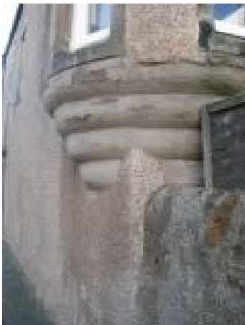
Modern dry dash render and cement slurry over sandstone masonry
