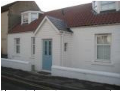
Upvc windows, doors, gutters and downpipes.
