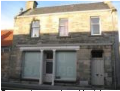
Former shop now in residential use
