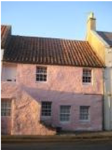
Stair House, Earlsferry
