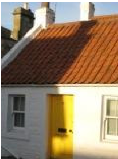
Modern brilliant white masonry paint and window frames, primary yellow door and orange painted pantiles.
