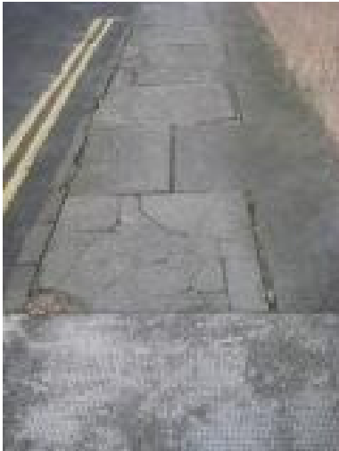
Concrete paving slabs and wet poured panels
