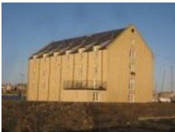
Warehouse, Elie Harbour
