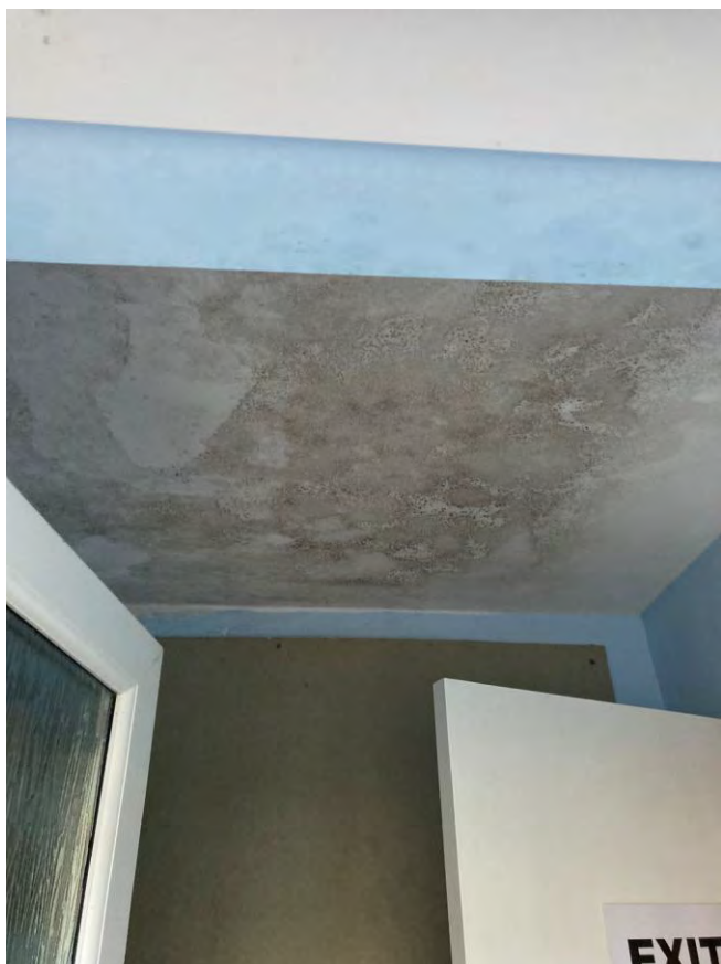
Water ingress due to failed porch
