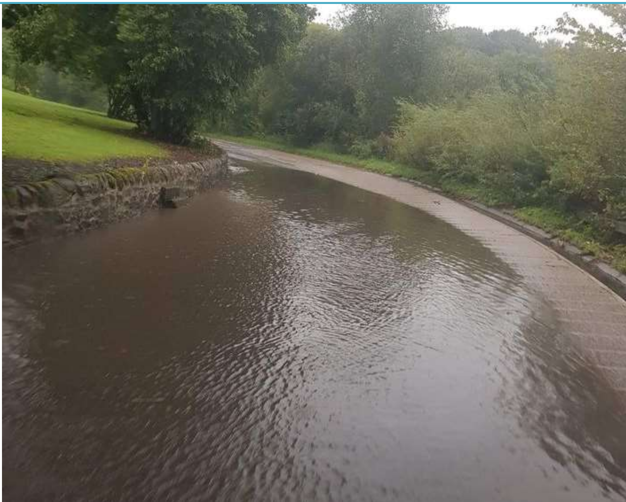
Figure 6. Flooding on Kinghorn Loch Road, August 2020
