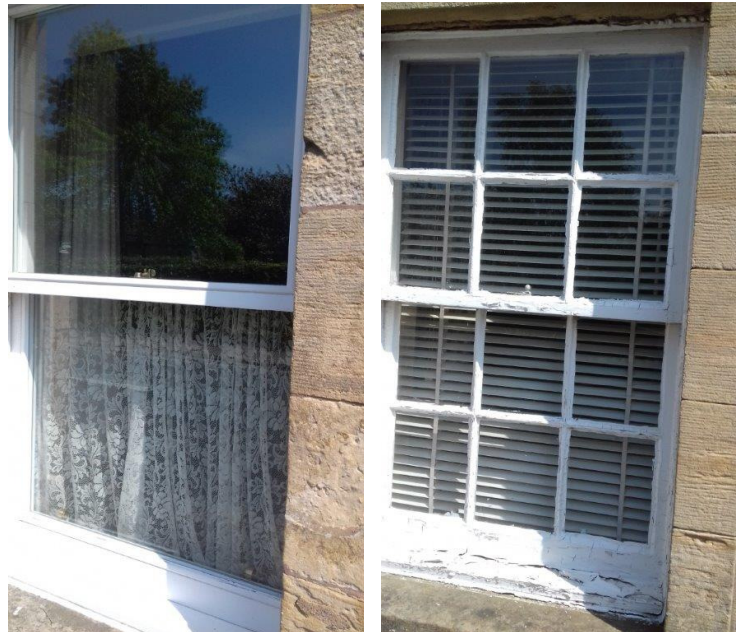
Contrasting glazing patterns – original right and modern replacement left.
