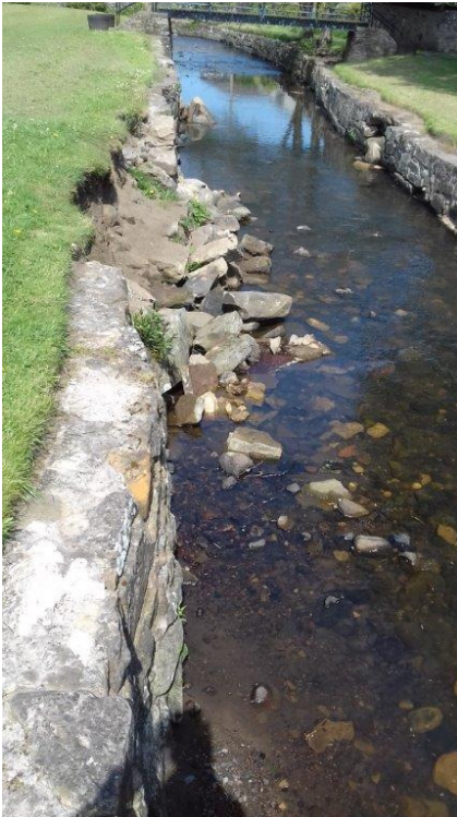
Ceres burn bank retaining walls.
