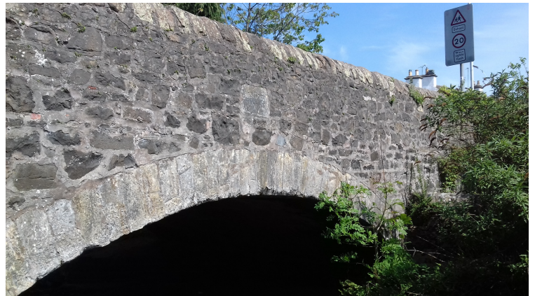
The 'new' 1831 Ceres bridge.
