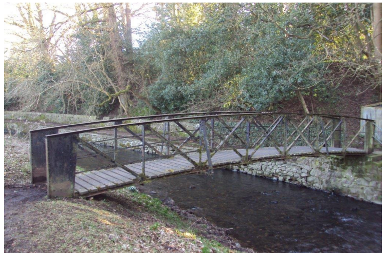
The footbridge and path to the south of Bow Butts.
