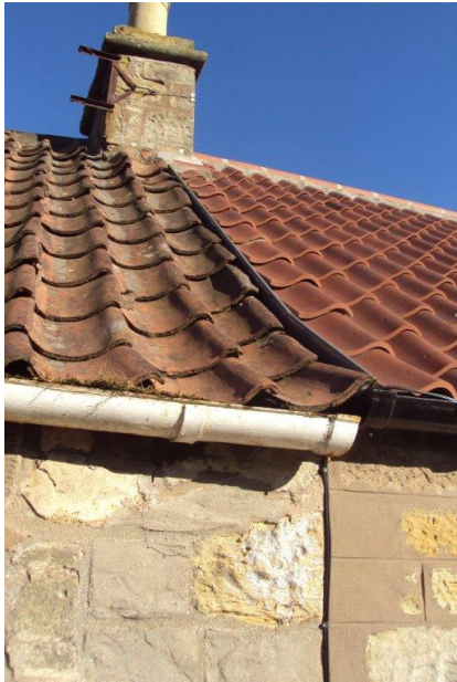
Renewed clay pantiles.
