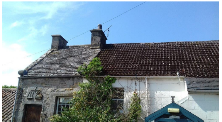
Contrasting traditional Scottish slates left with modern concrete tiles to right. The 1972 statutory list description only refers to pantiles.
