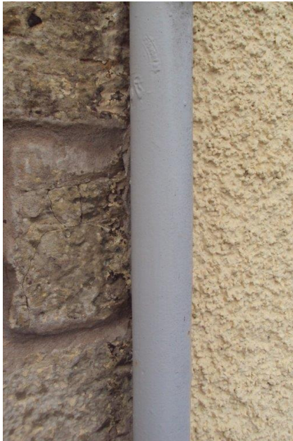
Modern cement render applied to a traditional listed weaver's cottage.
