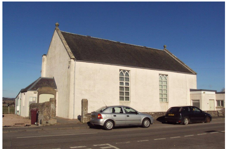
War Memorial Hall, Anstruther Road (above) Category B 1798 former Relief Meeting House.
