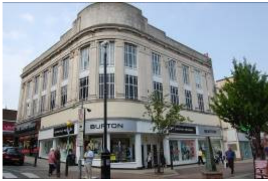
Burton's Building (built 1937)
