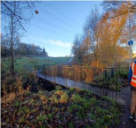
Bridge at Linburn Path heading towards Garvock Bank
