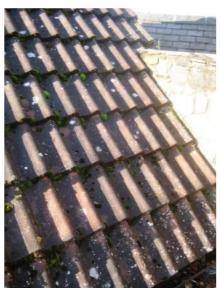
An example of inappropriate concrete roof tiles used on a building in the conservation area.
