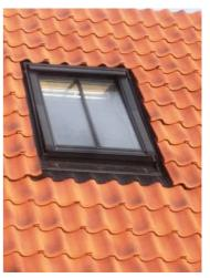
The basic design of the rooflight above right is similar to the traditional example above left. However, it is approx. 2.5 times as wide; with a dominant frame; and non-traditional apron material.
