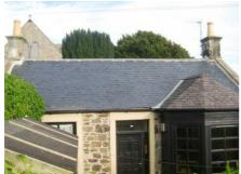
18 Schoolhill above originally would have been like adjacent 20 Schoolhill (below). Now has new roof slates and ridge tiles (was pantiled); inappropriate door and window style, colour and material; bay window added.
