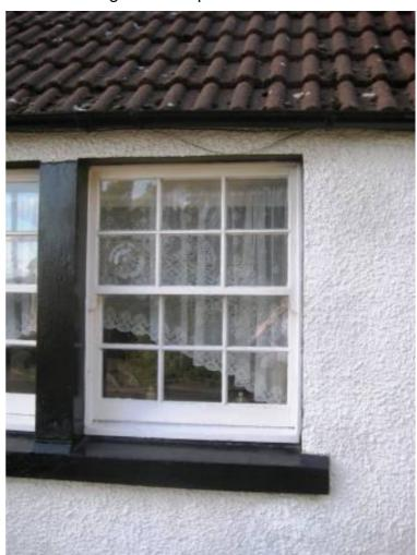
Example above: window detailing of 'horns', sill depth and crown glass all inappropriate for a building of this period and type.
