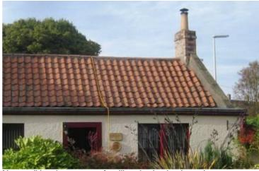
Non-traditional treatment of wallhead using lead capping.
