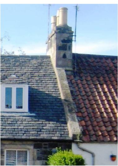
Characteristic features of Fife vernacular architecture – raised gable wall heads and red clay pantiles. Note: thackstane chimney head detail and 'blue' slates.
