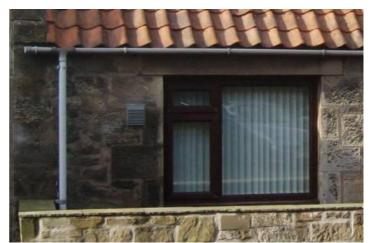
Enlarged window opening; stained dark wood frame; PVCu rainwater goods; new boundary wall with narrow cope; cement mortar pointing; vent grill.
