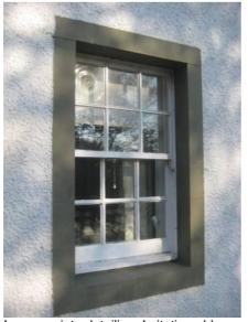
Inappropriate detailing. Imitation old Crown glass glazing in modern development. Note also non-traditional top sash horns.
