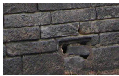
Missing ventilation grille
