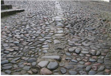
A sunken section of causeway paving is to be seen at the top of Mid Causeway near the Mercat Cross.
