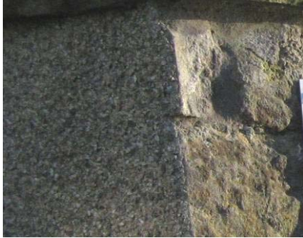
Example of dry dash applied to one face of rubble wall, likely to disrupt the normal processes of moisture movement through the wall
