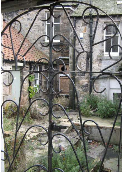
View of the back of the Dundonald Arms. Broken window panes, failing rainwater goods and growth of vegetation indicate decay as a result of being unoccupied.
