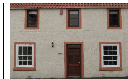
Replacement windows, uPVC, set far forward in the opening
