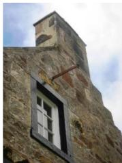
Above left -re-incorporated timber former fishing gear hoist gantry over a dormer window. Above right-unusual metal former fishing gear hoist gantry over a gable wall window.
