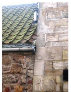
Rough rubble masonry left contrasting with snecked squared rubble right with its mixture of risers, levellers and snecks. Note characteristic traditional pantile roof with a slate easing course.
