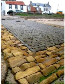
Harbour slipway constructed of whin setts with sandstone margin.
