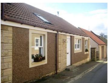
Traditional cottage with imitation stone cladding, dry-dash render, enlarged windows, PVCu door, modern sky-light, concrete roof tiles.
