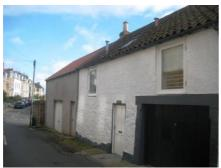
For example the significance of the traditional net loft dormer, including a hoist gantry, above left is diminished by the addition of a modern balcony; modern window and sky-lights and satellite dish. The chimney cans have also been lost. Note the different refractive characteristics of the original cylinder or crown glass compared to the modern float glass used to re-glaze the dormer.
