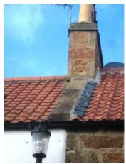
Examples of non-traditional skew cope detailing. Left-lead sheet encasing the gable skew cope. Right-row of slates over tile /skew junction.
