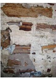
Above examples of the use of modern cement render on traditional sandstone rubble masonry (left) and pointing mortar (right).
