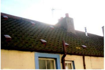
Conspicuous multiple modern vents on traditional pantile roof
