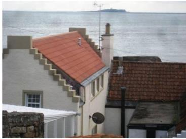
Contrasting imitation traditional roof left with authentic example right. Note reduced roof pitch, uniform tile form, colour and texture, narrow slate easing course width; enlarged proportions of gable steps; absence of chimney cans. And a satellite dish and TV ariel.
