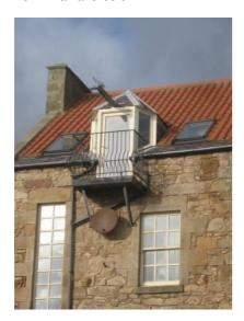
many of the 'dormers' are mid to late 19<sup>th</sup> century additions with, originally, associated hoist gantries inserted to provide access to the roof space sail lofts. Fixed external hoists were sometimes used for the nets, but sliding dormer beams were more common. Usually seen as a single central dormer per unit they were either designed as part of new houses or added to earlier ones during the mid-19<sup>th</sup> century herring fishing boom.
