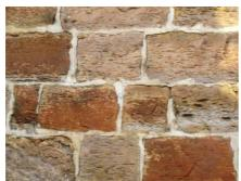
Example above of the adverse effect of cement mortar on masonry.
