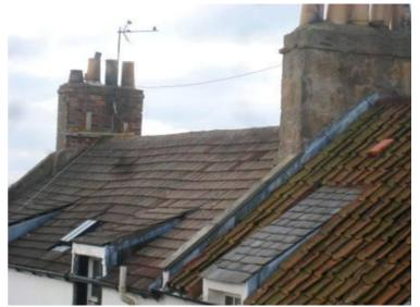
Modern concrete roof tiles on above left-hand roof. Contrast with traditional pantile roof to right.
