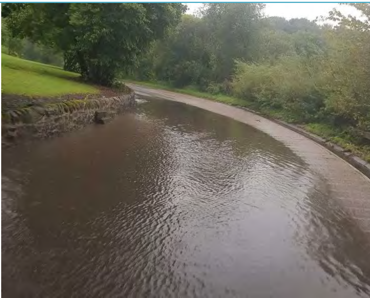
Figure 6. Flooding on Kinghorn Loch Road, August 2020
