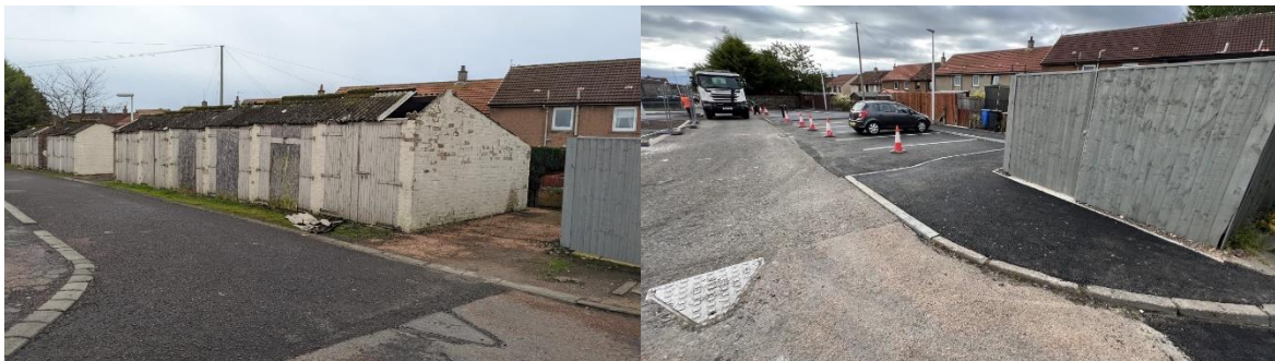
Cairnwell Place Lock Up demolition
