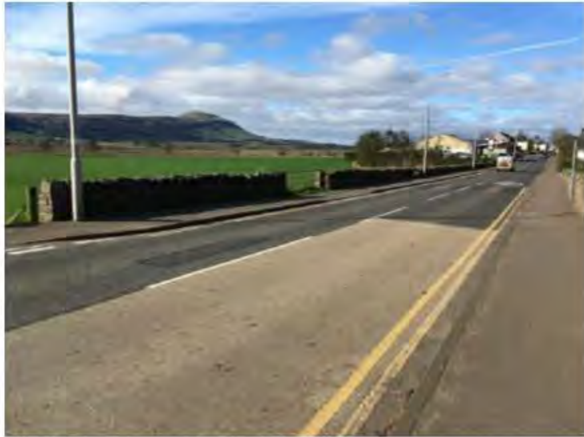
Photograph 1 – View along the frontage of the site (A91 Low Road)
