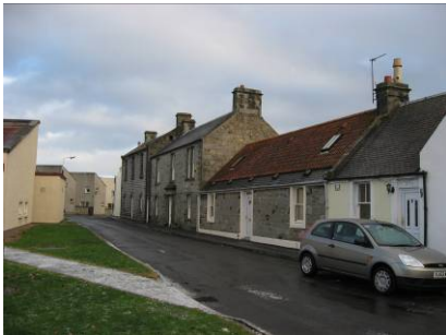
Different roofing materials on Forth Street; note the slated eaves margin to the pantile roof.
