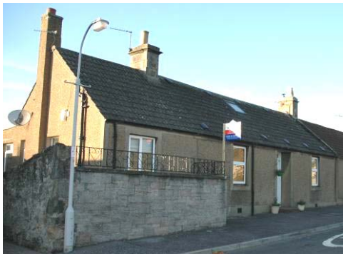
113-117 Kilbagie Street: concrete roof tiles, visible roof vents, cement dry dash walls, Upvc replacement windows & doors
