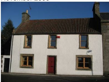
23 Forth Street photographed in January 2009. All windows replaced. Note change of ground floor to sash & case and loss of astragals to windows to upper storey.
