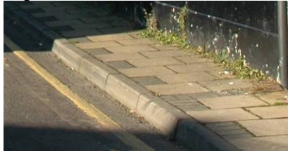
Excise Street pavement
