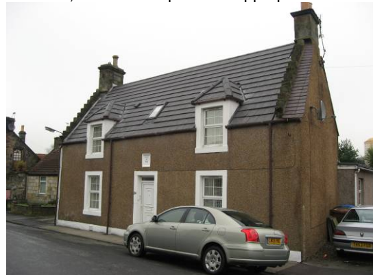
24 Kilbagie Street, B Listed: concrete roof tiles (installed Dec 2008), Upvc replacement windows and door, brown Upvc rainwater goods, satellite dish
