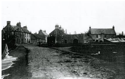
View of Keith Street from Shipping Pier c. 1900. (Courtesy of RCAHMS and Kincardine Local History Group)
