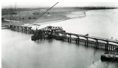
Forth Road Bridge under construction © Miller and Shepherd
