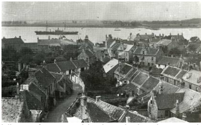
View of town with river in background, c.1920 before construction of bridge and North Approach Road © Miller and Shepherd
