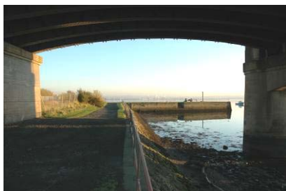
Shipping pier and promenade from north
