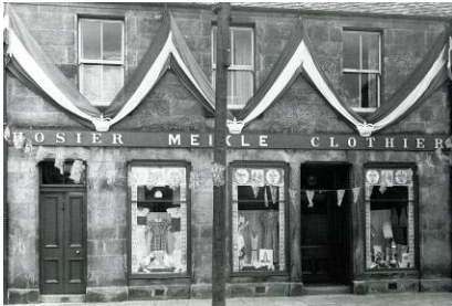
George Meikle's drapers shop on Elphinstone Street, 1952; painted timber sign is same size as stone band © Miller and Shepherd
