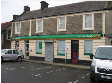
Channelled ashlar to ground floor, 22 to 26 High Street
