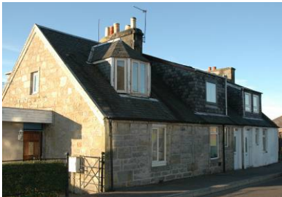
(L to R) 99-103 Kilbagie Street, poor design on RH houses, out of scale with cottages. Better to match original dormer to LH dwelling.
