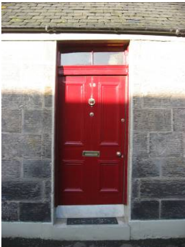
Panelled door with fanlight, Keith Street
