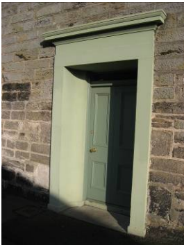
Recessed doorway on John Street
