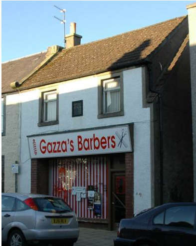
22 Elphinstone Street, C(S) listed: overlarge, unsympathetic shop sign and surround, non-traditional replacement windows, concrete roof tiles, chimney partially taken down
