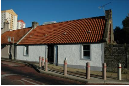
Traffic calming on Kirk Street
