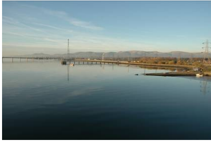
New Clackmannanshire bridge with Ferry Pier in foreground, December 2008
