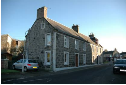
Rubble with dressed stone margins, 12 & 14 Kilbagie Street, note scroll skew putt
