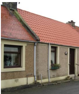
6 Hawkhill Road: Upvc rainwater goods
