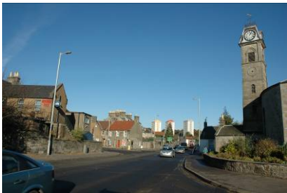
North Approach Road looking north; square in front of chapel now incorporated in to road
