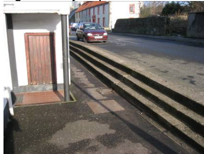
Kirk Street, in-situ concrete steps next to early C19 th building
