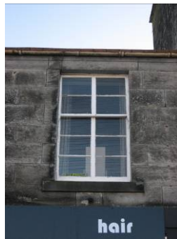
Timber sash & case window on High Street
