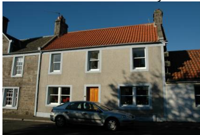
50 Keith Street, B listed, dry dash harling over original stone finish, bland in comparison to next door's natural stone
