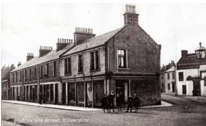
Elphinstone Street, dirt road with stone flag pavements. (Courtesy of RCAHMS and Kincardine Local History Group)
