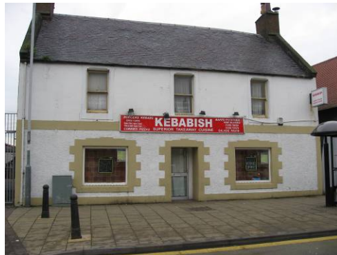
3 High Street: unsympathetic shop sign, non-traditional replacement windows & door to ground floor, wet dash to ground floor and non-traditional cement render surrounds to windows & doors
