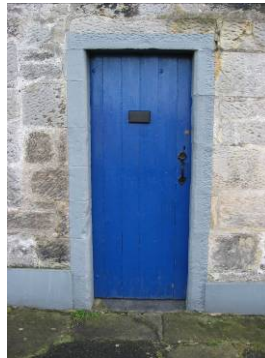
Timber ledged & boarded door, Forth Street
