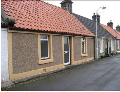
Replacement door and windows, Hawkhill Road
