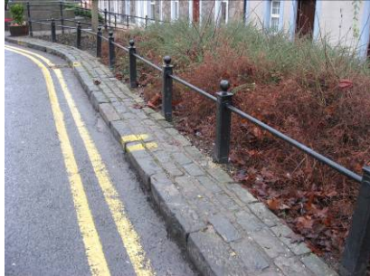
High Street, natural stone kerbs and setts around planting giving a softer edge
