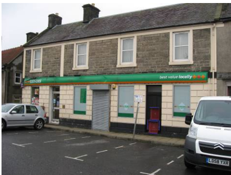
22 to 26 High Street, B listed: unsympathetic shop sign, non-traditional replacement windows & doors, inappropriate metal roller shutters
