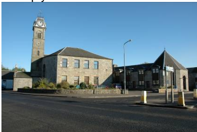
Low stone wall and planted border at flatted UP Church parking adds interest to street scene
