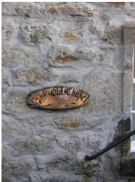
4 Cooper's Lane, B Listed, cement mortar pointing over stone face
