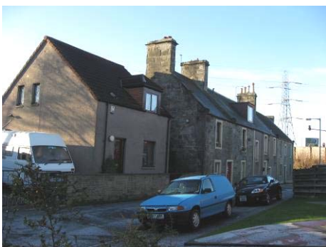
25 Silver Street constructed 1995: loss of street line and character as new property set back and 1½ storey not 2 storey as original neighbouring terrace
