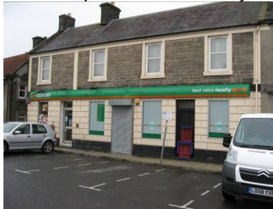
22 to 26 High Street, 2008, over large plastic shop sign concealing horizontal band
