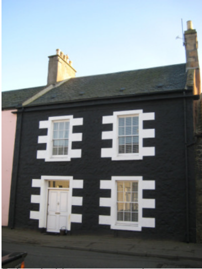
Painted whin masonry and upvc windows and door
