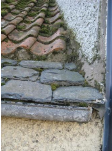
Typical traditional pantile roof with Scottish slate easing course
