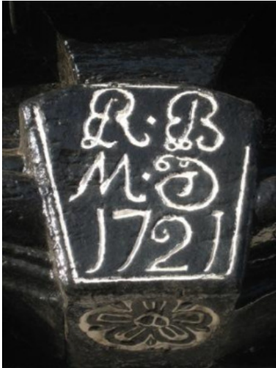
Dated key blocked doorpiece Commercial Inn, Main Street (rebuilt circa 1890).
