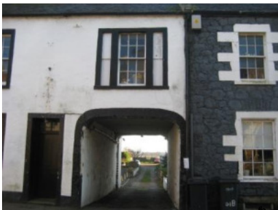
Former Balcarres Arms, late 18 th century coaching inn, Main Street. Note view through pend to fields beyond
