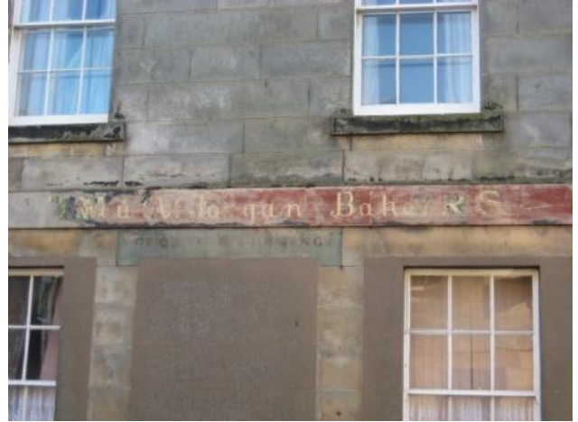
Example of original shop (bakers) sign. Blocked up shop door and reduced width windows
