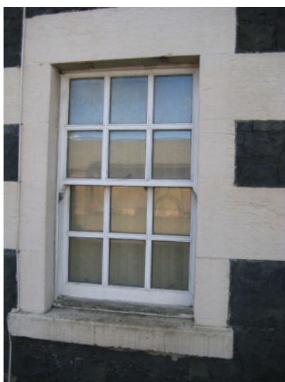
Upvc window with black glazing seals, enlarged astragals and incorrect detailing (horns).
