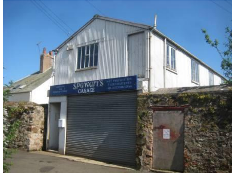
Corrugated iron clad building (modern roller shutter door)
