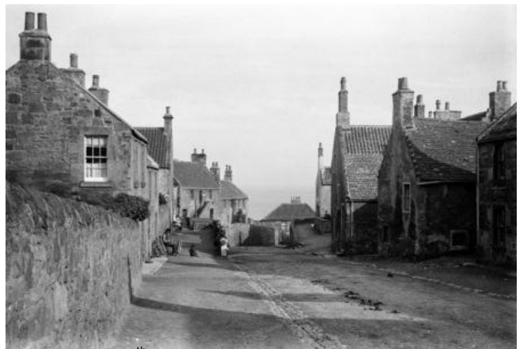
Shoregate late 19 th century . Note paved strip to first building on left. Source: CANMORE
