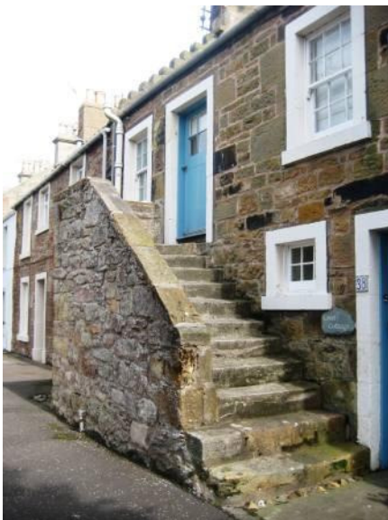
Typical fore stair feature.
