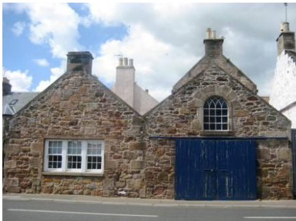
Past insertion of garage doors to a category C listed early 19 th century former school.
