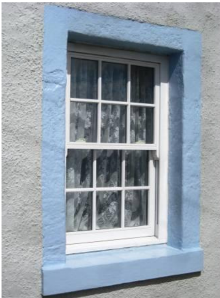
PVC-u double glazed windows with non-traditional 'horn' detail.
