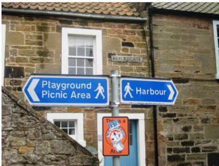
Signage detracting from category B listed building and conservation area. Note neglected traditional street sign.
