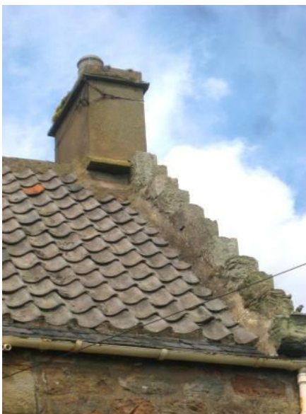
Re-built chimney head in brick and render but retaining thackstane detail.
