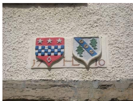
Cement render and modern film forming masonry paints can trap moisture and result in greater run off onto adjoining stonework. This can cause accelerated decay of stone beneath and adjacent.
