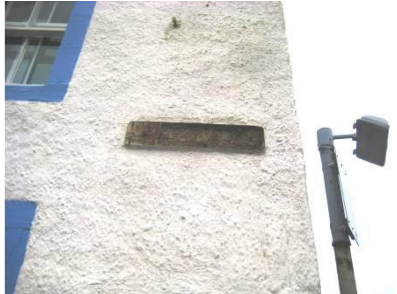
Missing signs on Kirk Wy nd.
