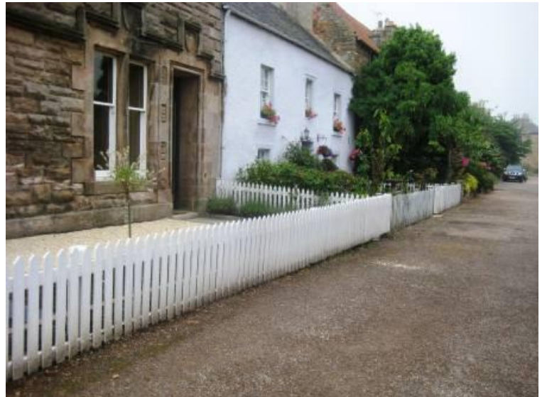
Stone chippings on Marketgate and simple low picket fence correspond with old photographs but not the brilliant white finish is not traditional.
