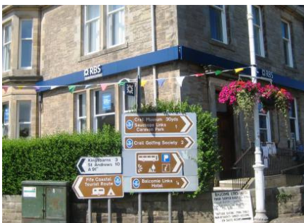
Signage detracting from listed building and conservation area as a whole.
