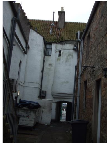
Rear of 42-43 Shore Street
