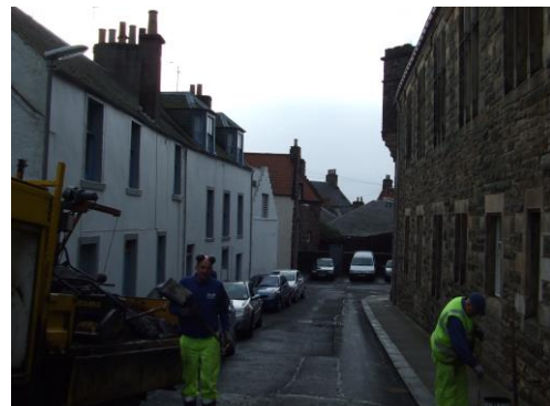
Patching historic granolithic paving on Kirk Wynd with tarmac – 2009
