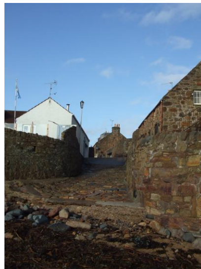
Slipway and seawalls at the foot of Crichton Street- 2009
