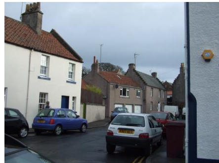
Satellite dishes, exposed cables, insensitively designed windows, cement renders, Cards Wynd - 2009
