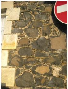
Whinstone rubble masonry with sandstone margins
