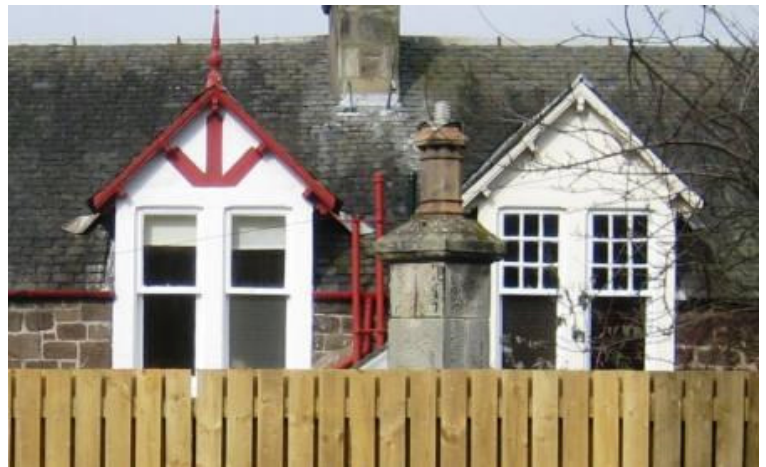
Above pair of windows were originally identical.
