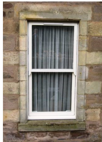
Replacement window above left was originally as the example next to it with six-over-six lying panes.
