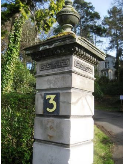
A functional though historically and architecturally inappropriate added house number.
