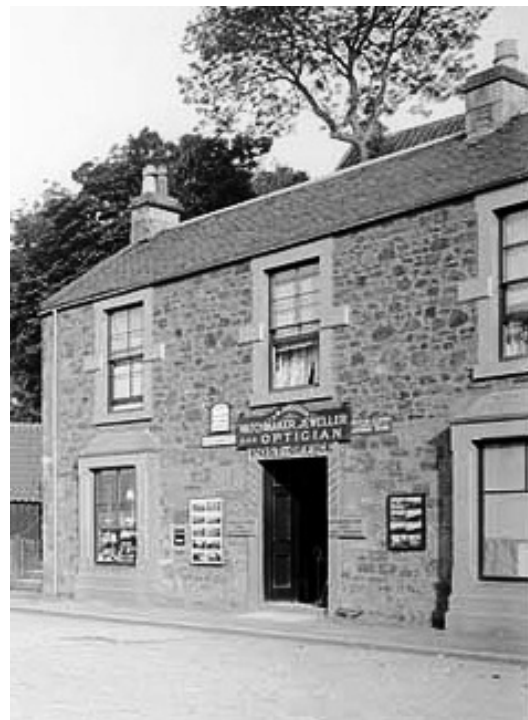
Typically dark painted window frames. Above example from early 20 th century photograph of Ferry Terminal.
