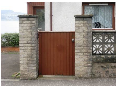
The modern gate piers and wall (above) contrast with traditional Victorian ones opposite (right).
