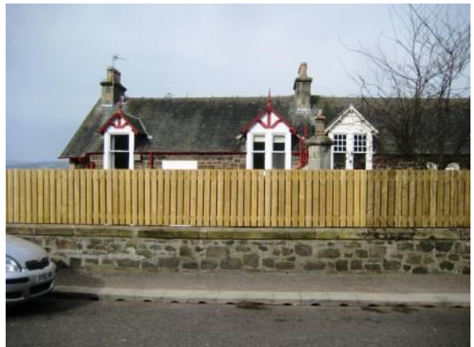
A modern style timber fence in place of cast iron railings.
