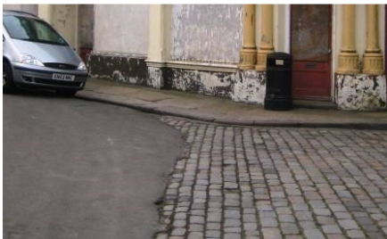
Early 19 th century sets at Ferry Pier, specifically noted as part of the statutory list entry.
