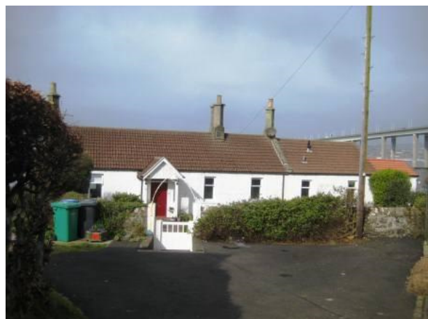
Modern concrete roof tiles on Craighead Cottage
