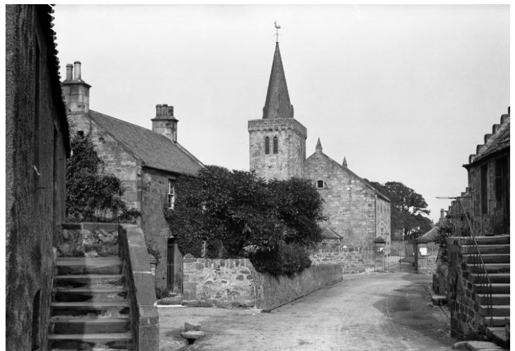
Main Street looking east early 20 th century and below now.
