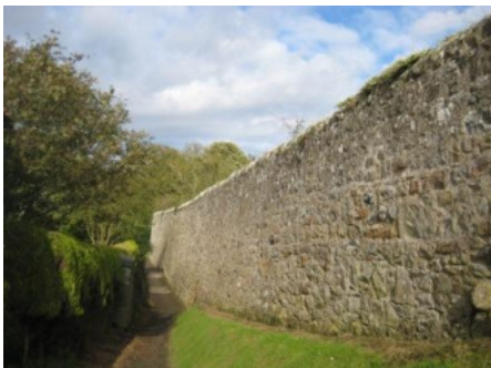
Rennyhill House boundary wall
