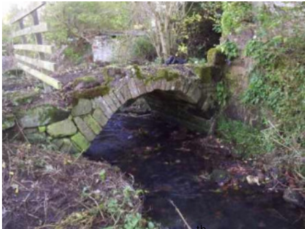
Kirk Wynd bridge – late 18 th century Category C listed
