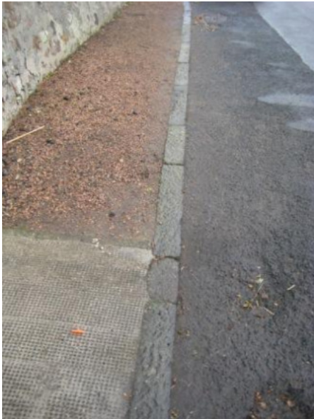
Modern road and pavement treatments.
