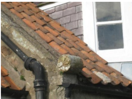
Scroll decorated (dog rose pattern) late 18 th century skew-put. Note dormer window addition.
