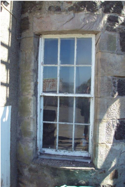
Historic glass in the stair window of a c1840 building.
