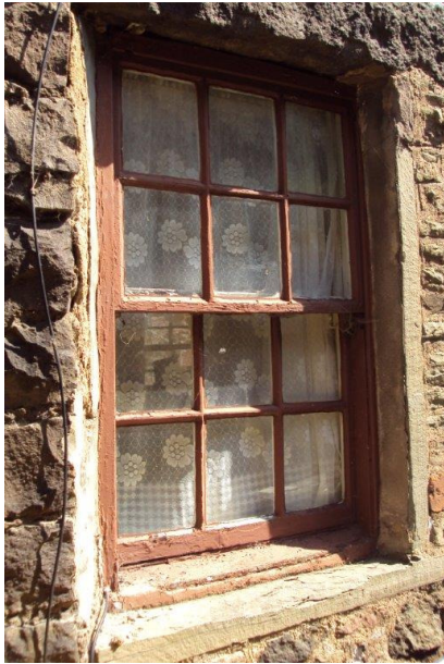
Typical Victorian sash and case window.
