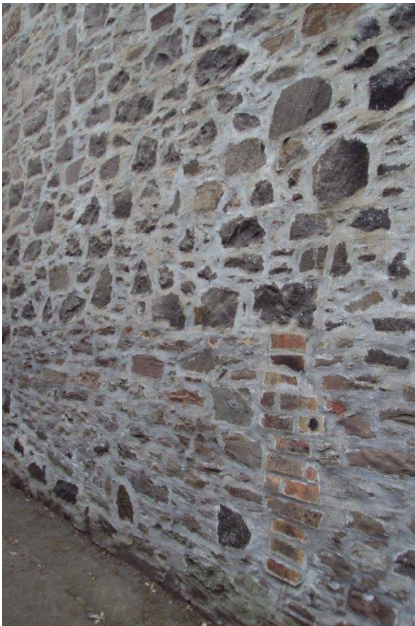
Cement mortar used for repointing.
