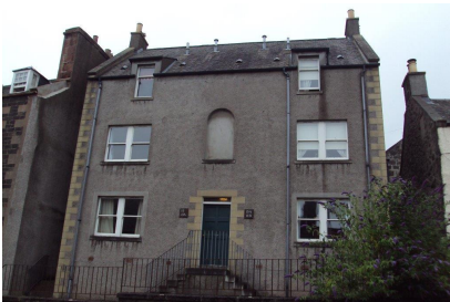
The above conversion and below new development have insensitive alien fenestration.
