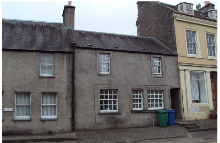
Contrasting original and replacement windows.
