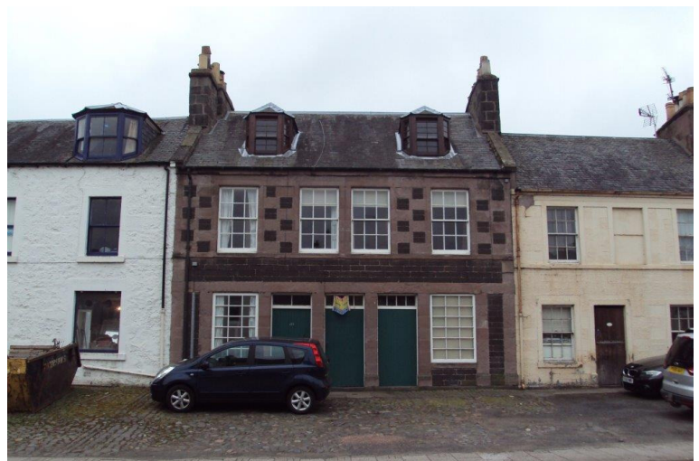
Contrasting dark whin masonry with lighter sandstone margins.
