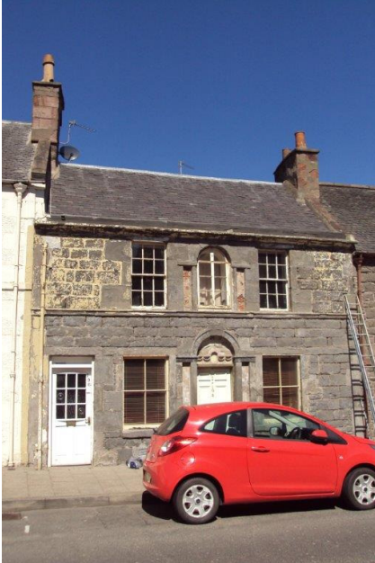
Above and below examples of Venetian windows and fore stairs. Above: 194 -196 High Street - late 18 th century
