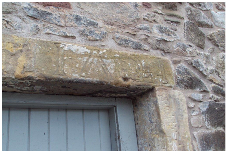
Removal of original stucco render.
