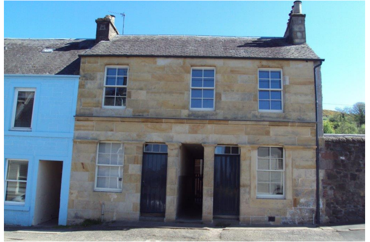
Paint removed from ashlar masonry.
