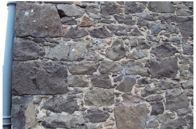
Original lime mortar pointing.
