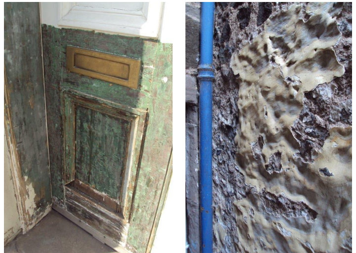
Evidence of former historic paint finishes and colours.
