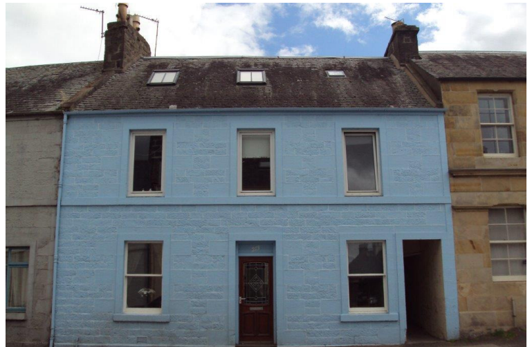
The above example shows the cumulative negative impact of multiple, relatively small scale, alterations and additions (i.e. inappropriate paint scheme; modern style windows and roof lights; modern style door).
