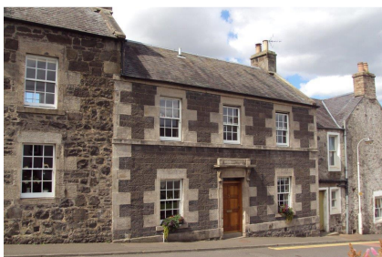
Typical style of building, materials and detailing.
