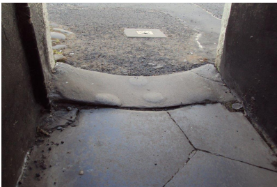
Above and below: stone threshold to a pend and paving showing the patina of time and wear.
