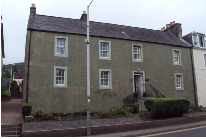
Example of a conversion showing some sensitivity to the vernacular architecture, although the additional bay unbalances the classic symmetry.
