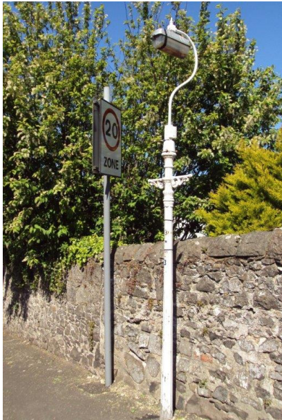
Historic street light column with later electric lamp addition.
