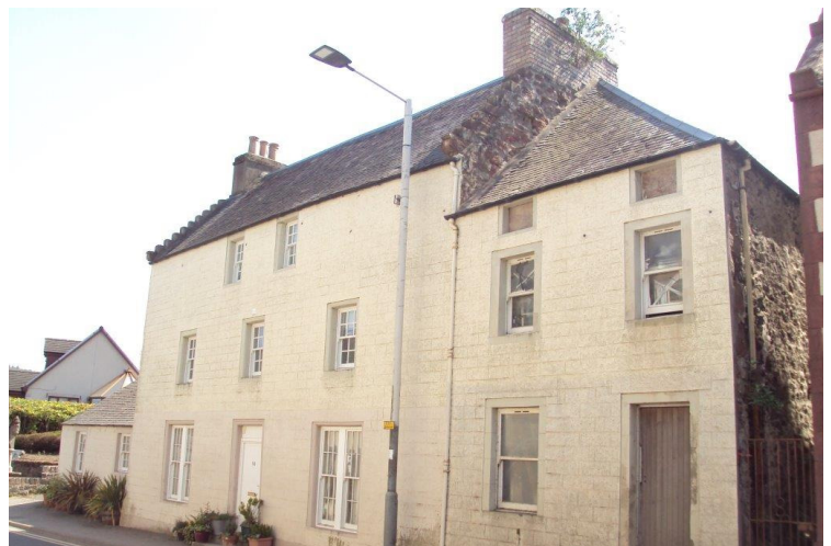
'Restoration in Progress' at 1-3 High Street
