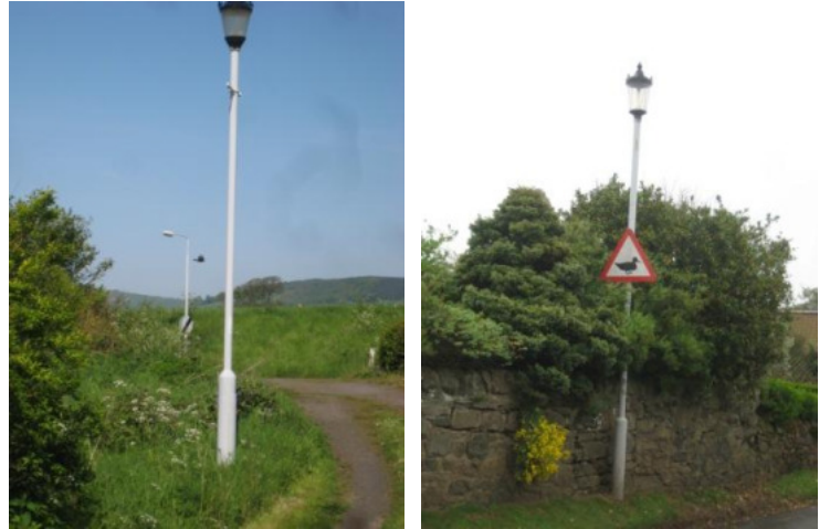
Example of the inappropriate style of street light used throughout the conservation area
