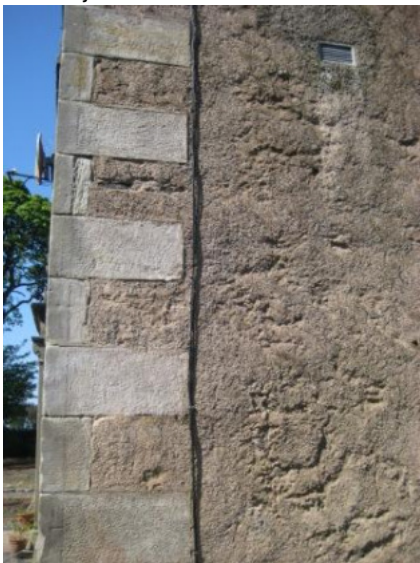
Example of typical traditional lime harled rubble masonry
