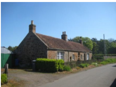
Alexander Cottage, Greenbrig Road
