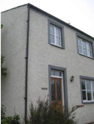
New development on the site of a listed building, in a prime location next to kirk – similar proportions, footprint and orientation but cement dry-dash render; plastic rainwater goods; upvc windows; varnished, glazed door; and a carriage lamp
