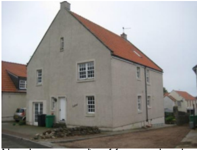
New house on site of former church and more latterly village hall – similar footprint, orientation and proportions but architecturally out of character
