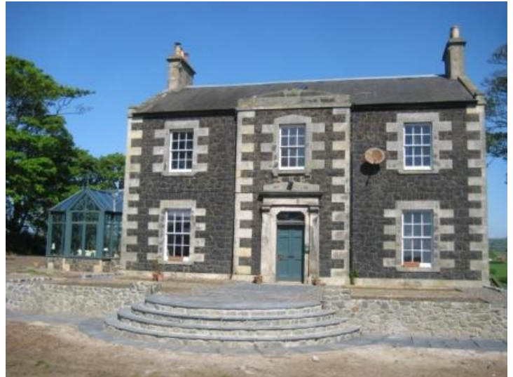
Satellite dish on Category B listed former Parish Church Manse, Kilconquhar
