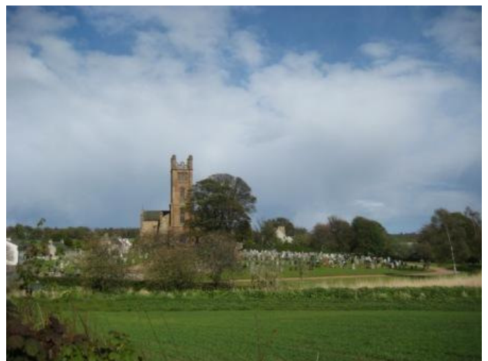
Kilconquhar Parish Church knoll dominates the conservation area
