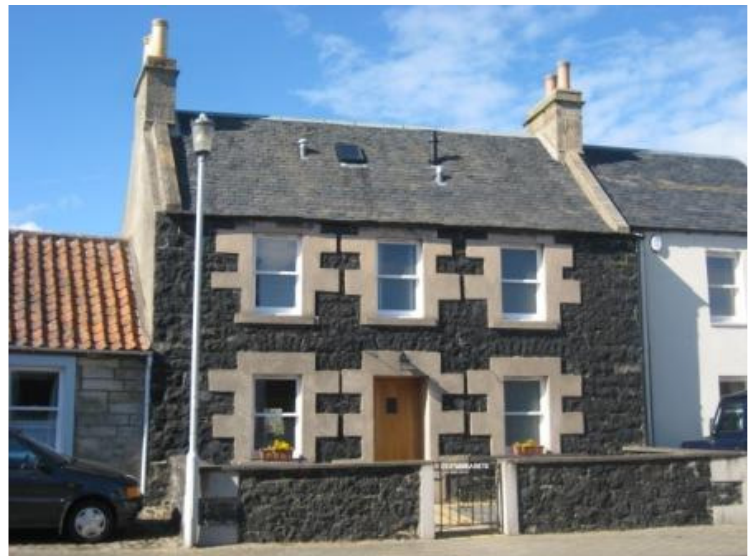
St Margaret's 41 Main Street – an attractive blue whinstone masonry façade with distinctive traditional 'cherry-cocking', marred by cement door and window margins. Also note inappropriate varnished 'cottage' style door, concrete wall cope and plastic flues through roof.
