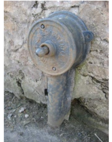
Left above: Charter bole in car park wall with 13 Main Street. Right above: Cast iron stand pipe attached to kirky ard wall on Main Street. Manufactured by Glenfield & Kennedy, Kilmarnock. Patented 1902 and used up to 1950. There are two other similar examples along the Main Street.
