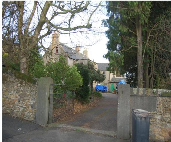
*Hard cement has been used here to repair gate piers, which will cause the stonework to deteriorate over time*
