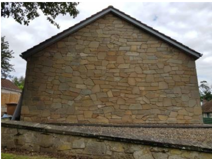
Incongruous crazy-paving style face-bedded stone cladding.
