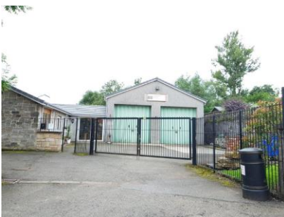
Modern light industrial unit and yard occupying site of former maltings.
