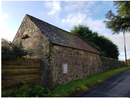
Building adjacent former dairy Monimail Road
