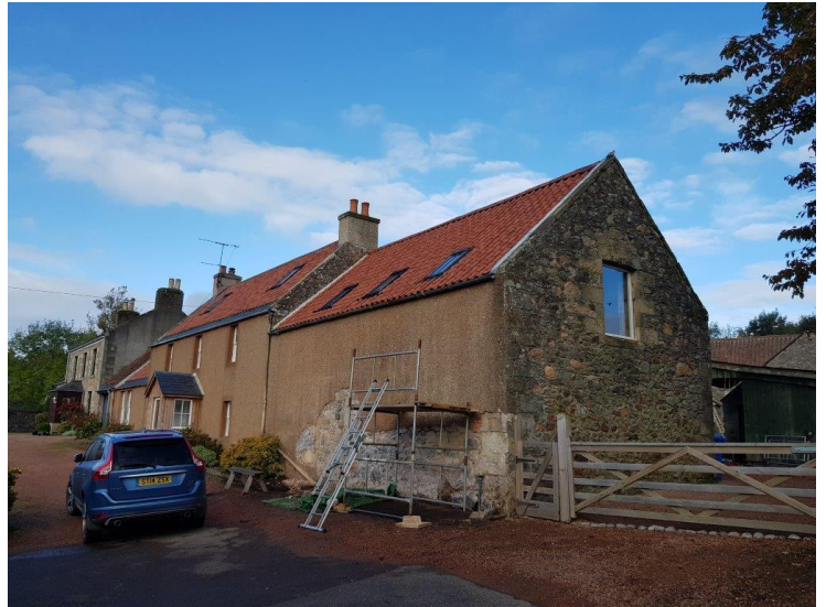
Modern cement render removed to reveal the original masonry.
