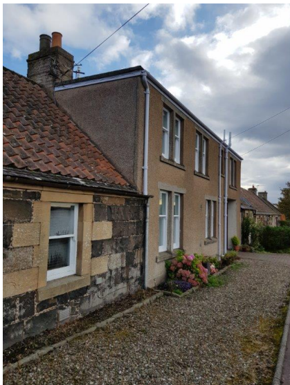
Past unsympathetic first floor extension.
