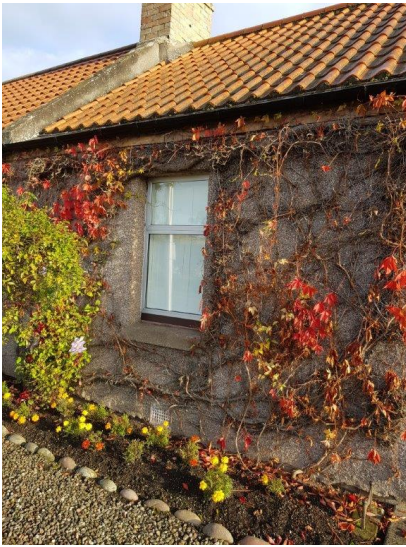
Non-traditional aluminium window frames.
