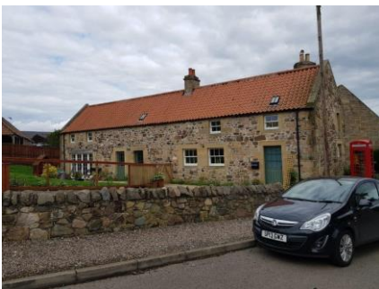
Alterations to adapt the above for residential use have changed its character.
