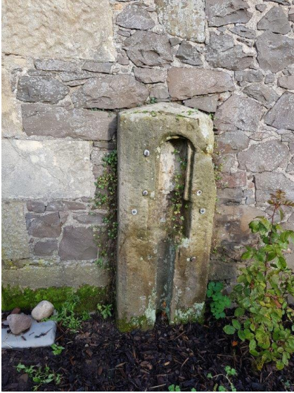
Typical random rubble masonry. Note housing for former water pump shown on 1854 Ordnance Survey map.
