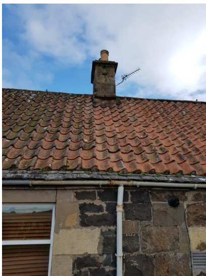
Typical examples (above and below) of pantiled roofs on, probably, originally thatched buildings. Note thack stanes.
