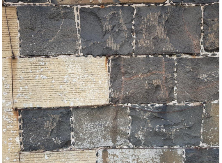
Squared coursed whin masonry with decorative cherry caulking; contrasting with droved pale sandstone ashlar rybats.
