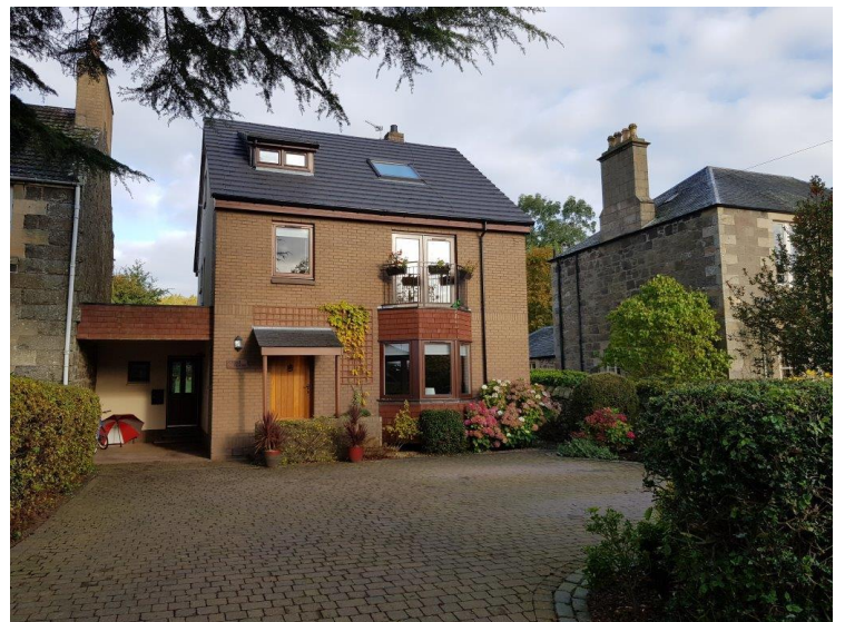
Modern infill with incongruous materials and architectural paradigms.
