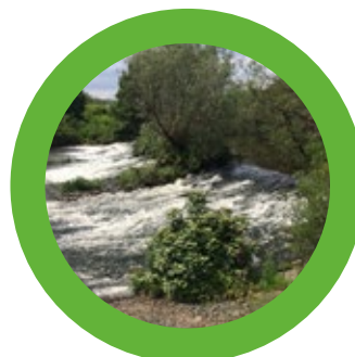
River Leven Burn Mill Weir
