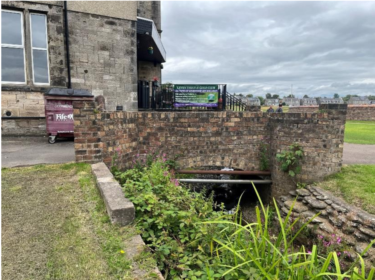
Figure 3: Leven Thistle Clubhouse Bridge with exposed common brickwork
