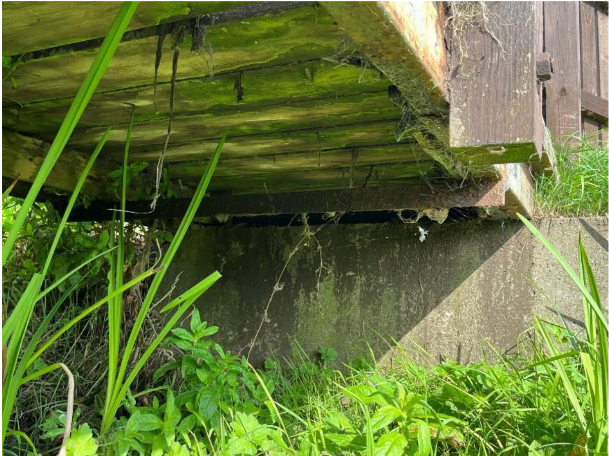
Figure 6:Underside of existing deck and abutment
